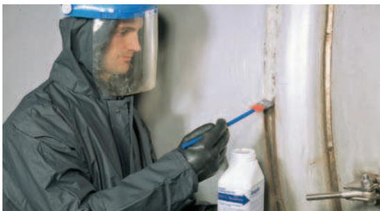
Avesta Pickling Gel 122 is easy to apply thanks to its free-flowing consistency.
